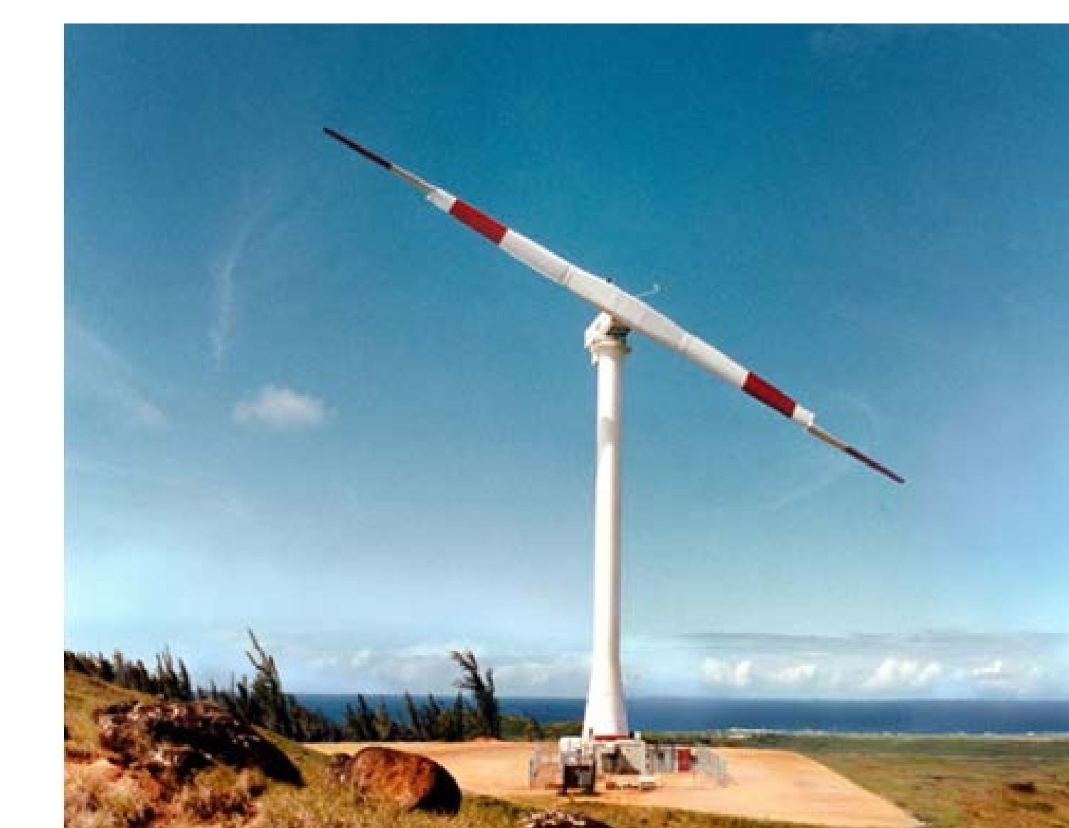
MOD-5B Wind Turbine (Two-bladed, teetered hub, 3.2 MW)
